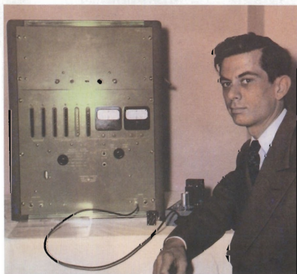
In 1951, Al Bagley's development of HP's new 524A high-speed frequency counter reduced the time needed to measure high frequencies from minutes to seconds.
